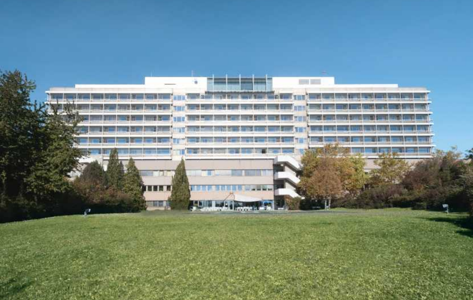
Leopoldina Hospital in Schweinfurt has a drinking water installation system featuring components from Georg Fischer JRG.
